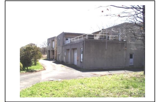
Liquid waste treatment facility
