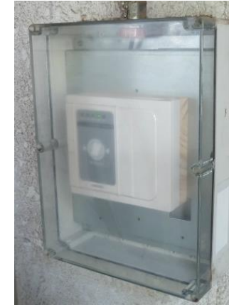
3 F Entrance near the stairs
